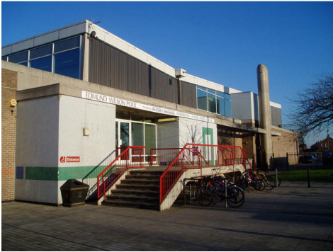
Image 4.3 The replaced Edmond Wilson Pool
