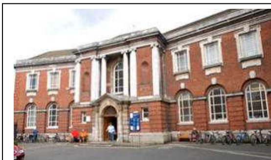
Image 5.1 Exterior of York Library
